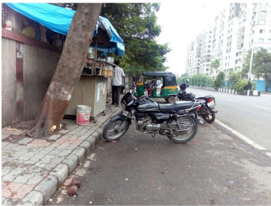
11-CONDITION OF FOOTPATH.jpg
