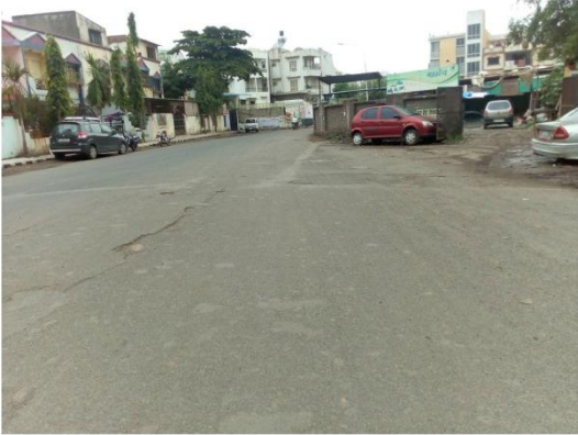
01-CONDITION OF CARRIAGEWAY.jpg
