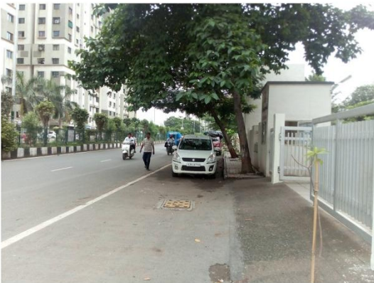
03-STORM WATER DRAIN.jpg
