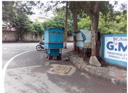
06-TREE ON FOOTPATH-OBSTRUCTION.jpg
