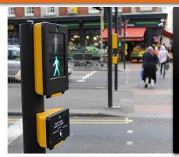
"Push to talk having audible signals installed at Pedestrian Crossing specially for Children, Elder & Handicapped. It may also be installed on Smart Pole."
