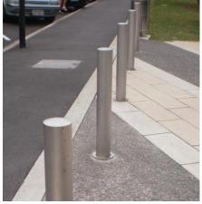
Provisions for Handicapped: First Image shows ramp provision for public transport, second image shows proper slope/ramp to get on road comfortably & third image shows bollards having min. spacing 1.2 m.
