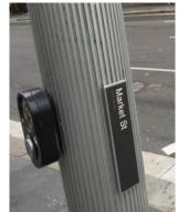
**Provisions for Blind:** First Image shows tactile paving for direction guidance, second image shows braille signage/way finding & third image shows push to talk with braille signage and audible signal.
