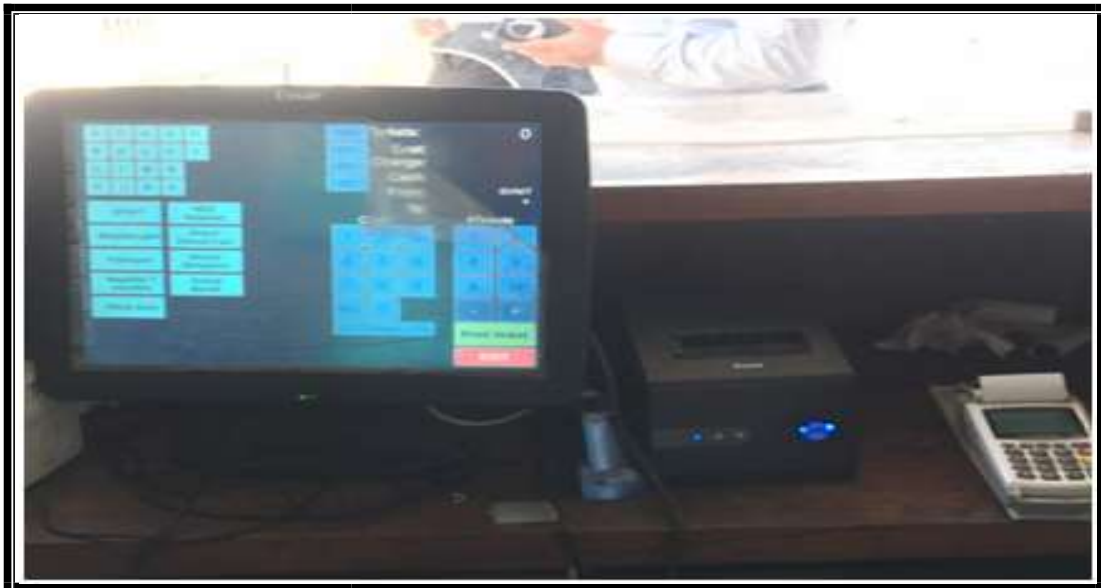
POS Machine at BRTS Stop
